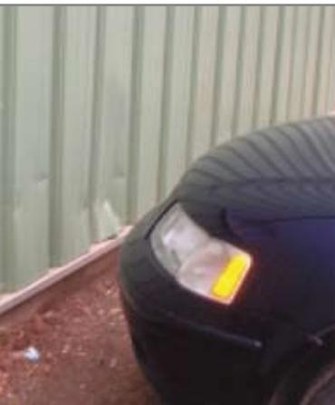
*Steel cladding dented by parking cars.*
